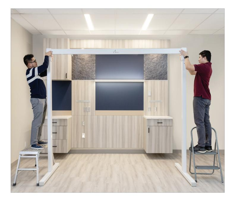
Once the track assembly is properly placed onto the two posts, ensure that the mounting holes and the track assembly is aligned. Fasten the 3/8" socket cap screws on both sides to properly secure the track assembly to the posts.
