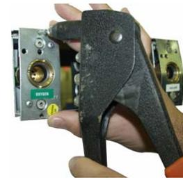
A filler frame is placed over the conversion to hide any gaps and allow correct spacing from the outlet backs to the outlet fronts (this is like a gasket).
