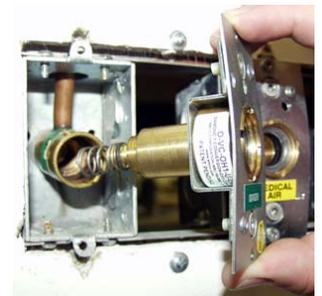
Screw Diamond 1 conversion into rough-in body with the conversion tool.
