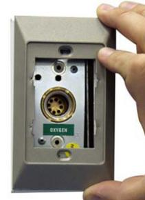
The Amico latch valve is then placed over the frame and sandwiches the whole assembly together with the latch valve screws.
