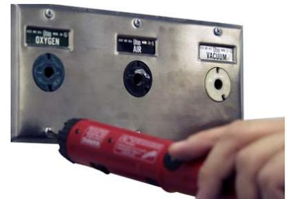
Remove all internal components so that the threads in the back are exposed.
